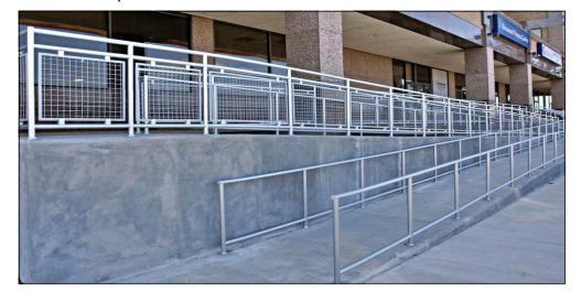
To avoid these problems, HMS selected Hollaender's® anodized aluminum Interna-Rail® railing system with electro-coated/powder coated steel wire mesh infill panels. The anodized aluminum withstands pedestrian traffic much better than painted steel, and both the aluminum railing frame and the e-coated/powder coated panels resist corrosion better in the Gulf of Mexico coastal environment.
