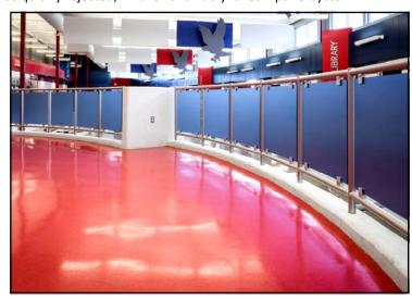
Joe found that Hollaender® Manufacturing's Interna-Rail® anodized aluminum railing system, combined with Lumicor® Lago acrylic resin infill panels offered the school the look and functionality they wanted, at a price they could afford. In addition, all involved liked the fact that Hollaender's component/non-welded design gave it a versatility that was an added feature.
