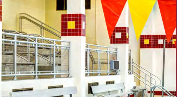
Interna-Rail® with Stainless Steel Wire Mesh Infill Panels
