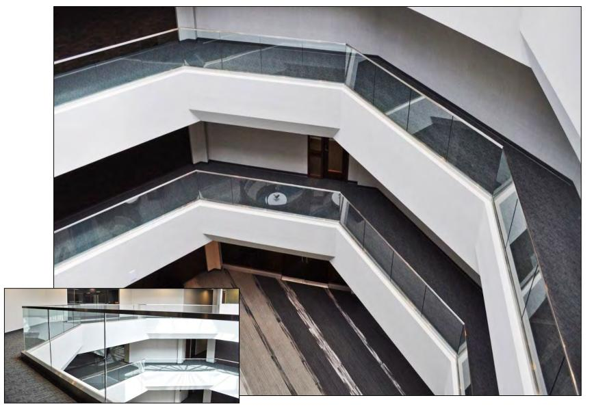
Stainless Steel Cladding and 2  $\frac{1}{2}$ " Top Cap with  $\frac{1}{2}$ " Monolithic Glass
