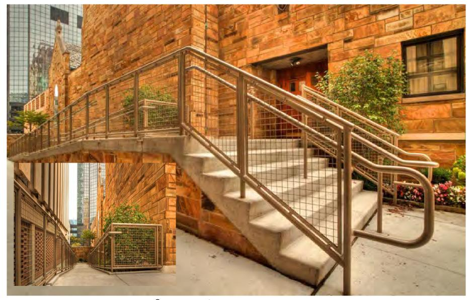
Interna-Rail® Powder Coated with Wire Mesh Infill Panels
