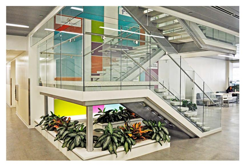
Coated Aluminum Cladding with Stainless Steel Assist Rail
