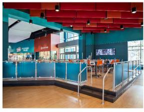
Interna-Rail® Aluminum Railing System Clear Anodized with Acrylic Infill Panels
