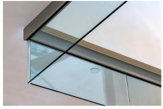
**SMOKE BAFFLE**Clear Tempered Glass
