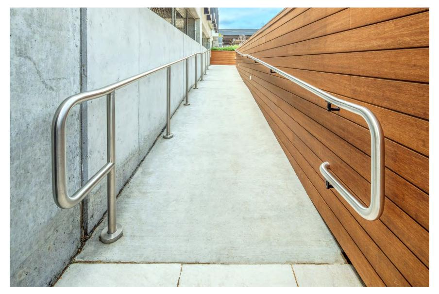
**Stainless Steel ADA Compliant Handrail**
