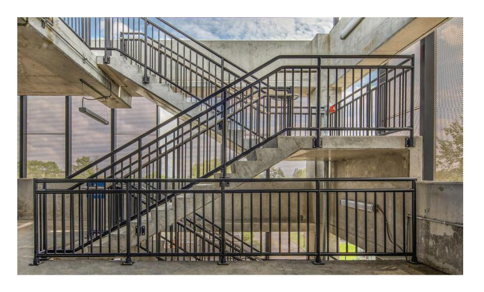
Interna-Rail® Aluminum Railing System Black Anodized with Pickets
