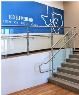
Stainless Steel VUE™ Railing System with Glass Infill
