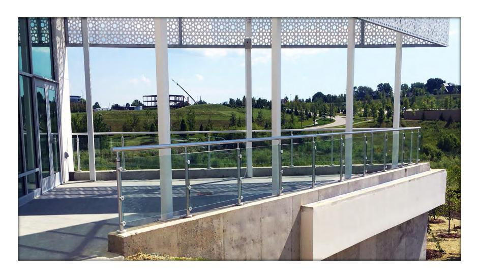
**VUE™ Clear Anodized Railing System with Glass Infill**
