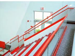
STRUCTURAL GLASS WITH CLEAR TEMPERED INFILL PANELS
