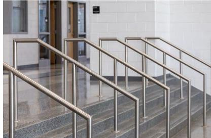
STAINLESS STEEL POST AND WALL MOUNTED HANDRAIL
