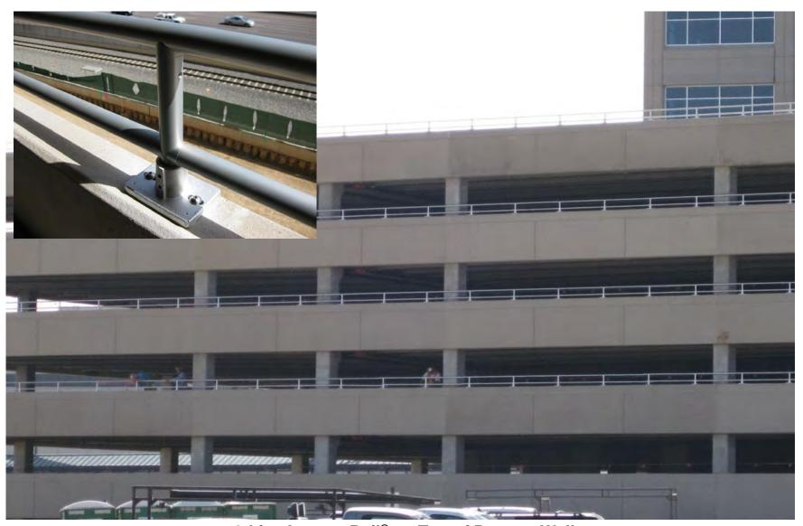
**2-Line Interna-Rail® on Top of Parapet Wall**Village Center Parking Garage *Denver, Colorado*
