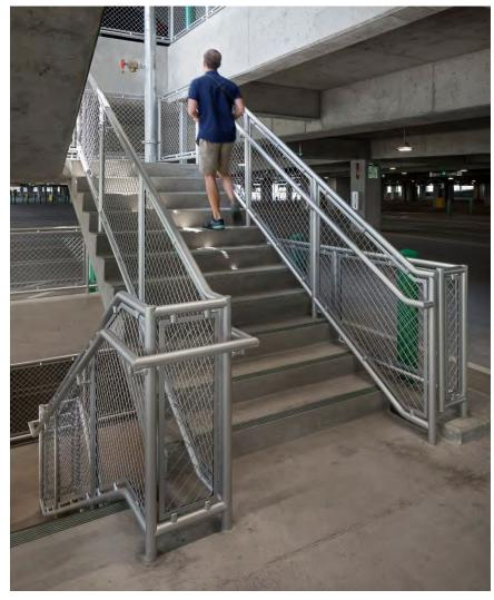
Interna-Rail® Aluminum Railing System Clear Anodized with Diamond Wire Mesh Infill
