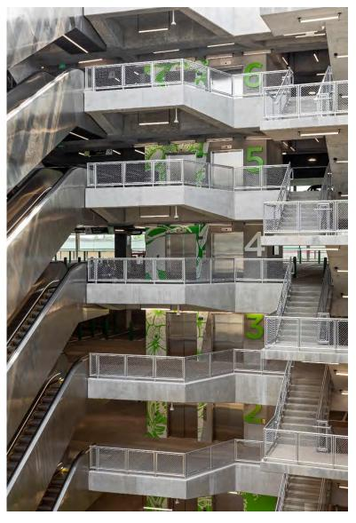
Interna-Rail® Aluminum Railing System Clear Anodized with Diamond Wire Mesh Infill
