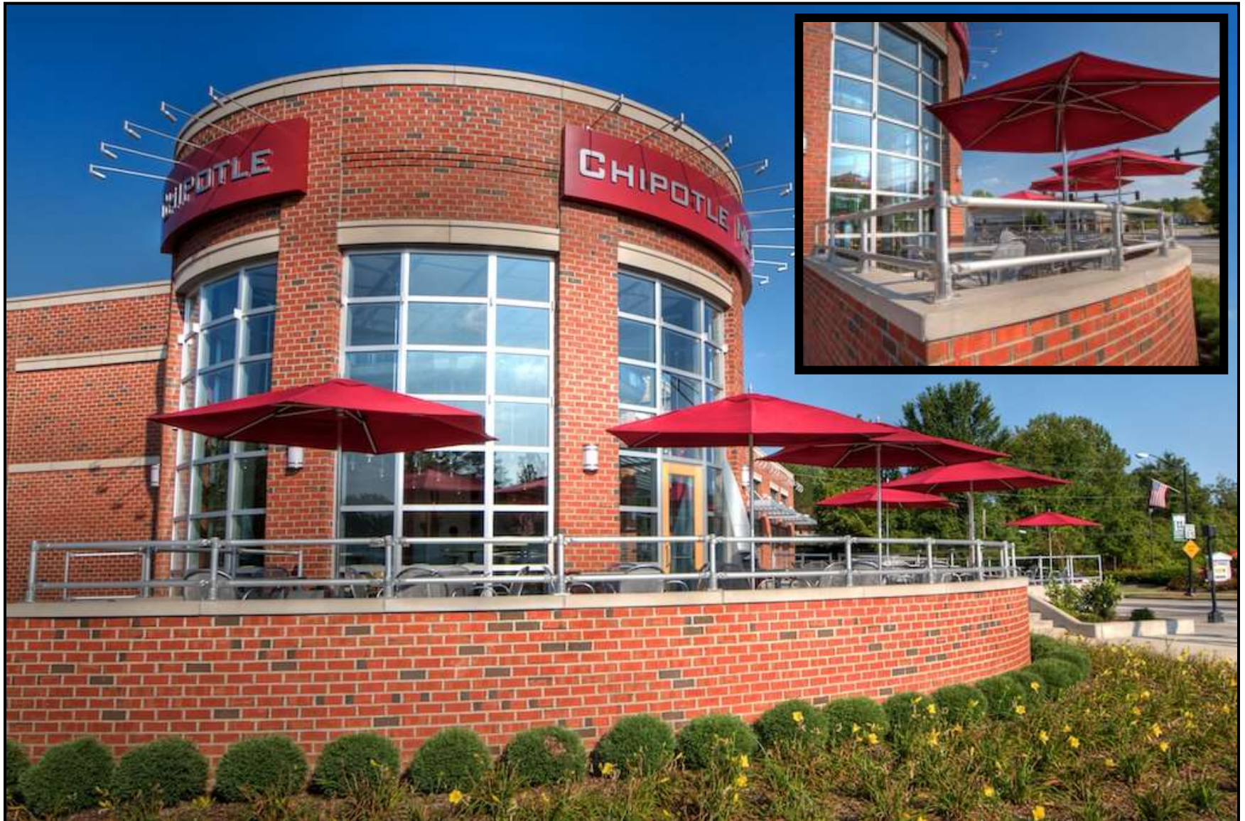
CHIPOTLE - Speed-Rail® Application
