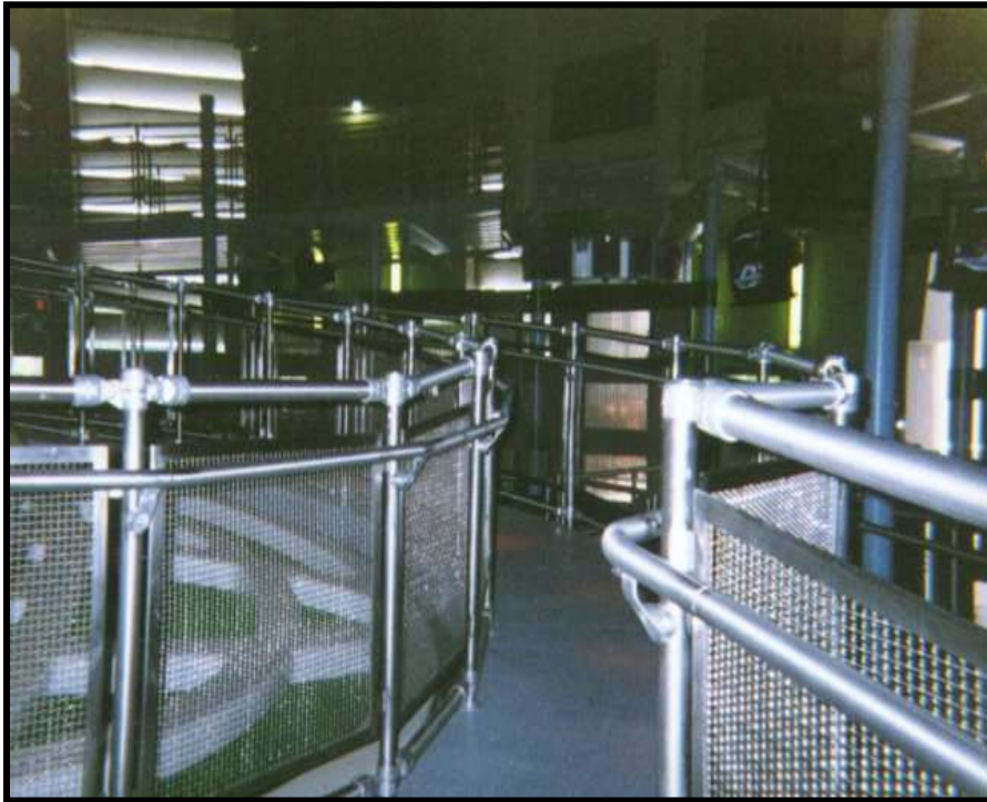
ADA System with OSHA guardrail and infill panels.
