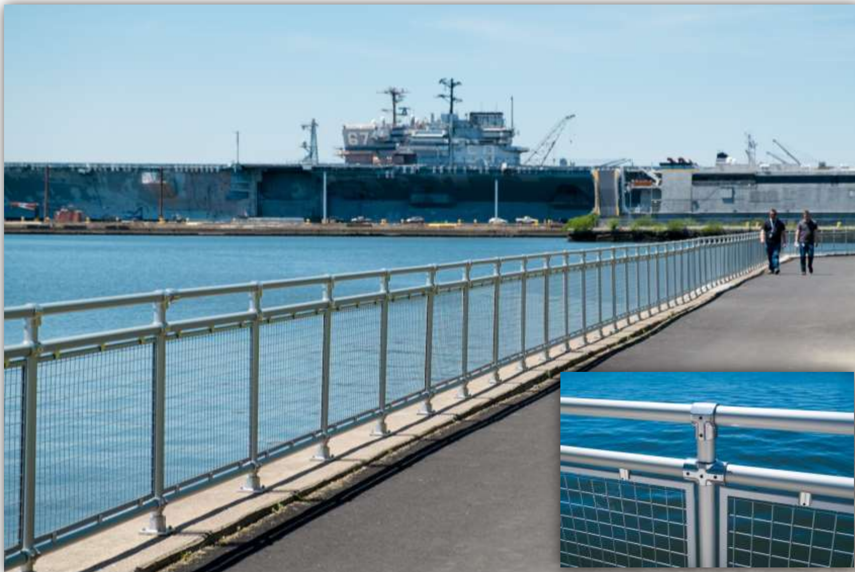
Speed-Rail® with Wire Mesh Infill Panels Philadelphia Naval Shipyard
