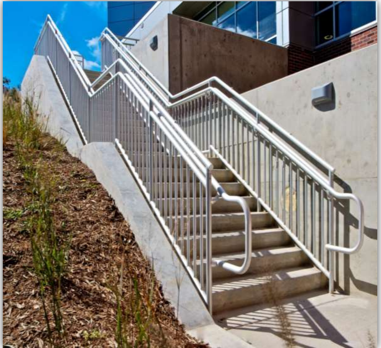
ADA Handrail Clear Anodized with Picket University of Nebraska – Omaha Campus
